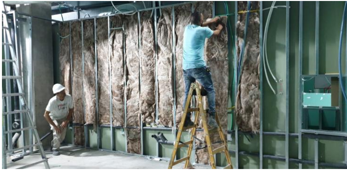
Gypsum wall & insulation
