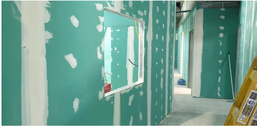
Gypsum wall & insulation
