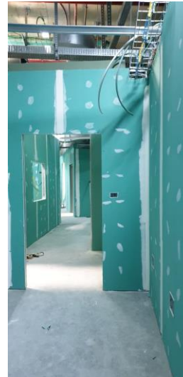
Gypsum wall & insulation
