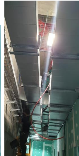
Continuing above ceiling works
