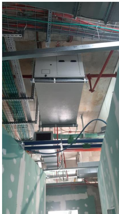
HVAC equipment installation
