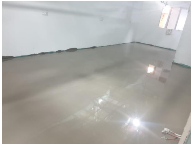
Cement self-leveling flooring
